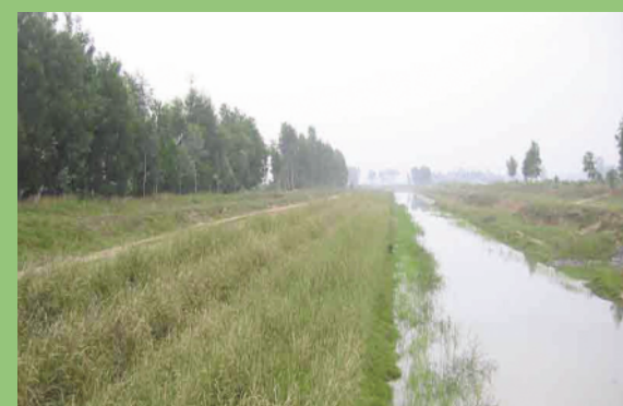
Vietnam - the left hand bank of the canal has been reshaped and stabilized with vetiver, the right bank has yet to be treated.
