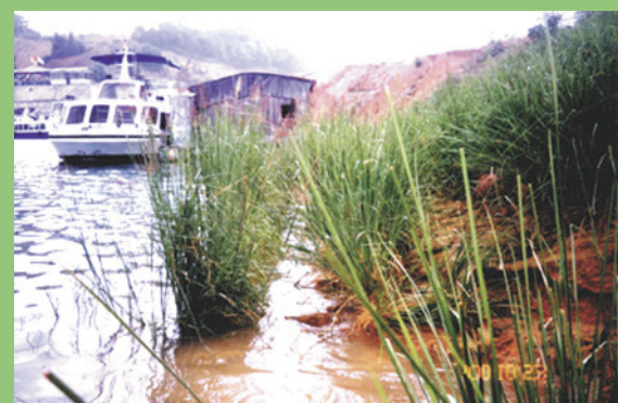
China - partially submerged vetiver grass used to stabilize the draw-down slope of a reservoir in Guangdong Province
