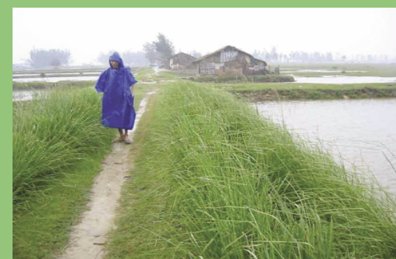
Vietnam - cyclone damage to sea dykes is a major problem. VS has been applied successfully for disaster mitigation
