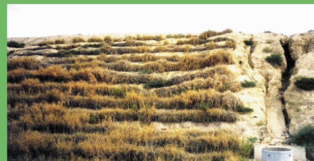
Spain - unstable and eroding highway fill treated with VS. Untreated eroded fill on right. VS grows well under low rainfall Mediterranean climate
