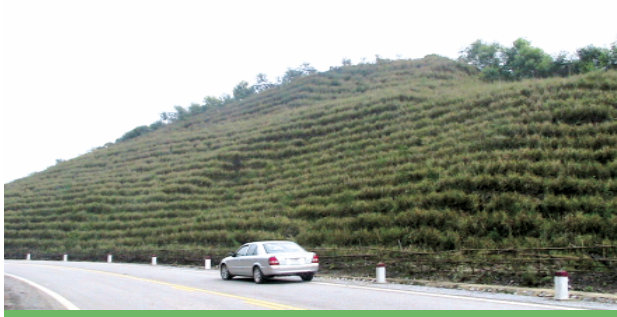
Vietnam: the Ho Chi Minh Highway has been stabilized with vetiver grass. The batters and fills are stable and withstand cyclonic rainfall events
