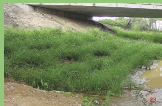
Australia - this river bank and bridge abutment have been stabilized with vetiver. Vetiver is an excellent interface for concrete and soil
