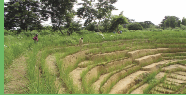
Congo D.R. - huge gullies that destroy urban areas and houses can be rehabilitated and stabilized using the Vetiver System.
